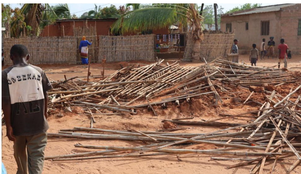
Completely destroyed house by Cyclone Chido @IOM 2024/Gerson Fanequico
